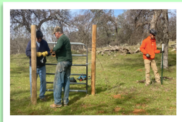
GCTC members Jeff Foltz and Jerry Gridley, along with a PLT volunteer, working on installing Kiwi-Style Chain latches and replacing barbed wire with barbless wire near gates.
